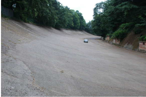
Surviving Section of Brooklands Banking with MGB GT
